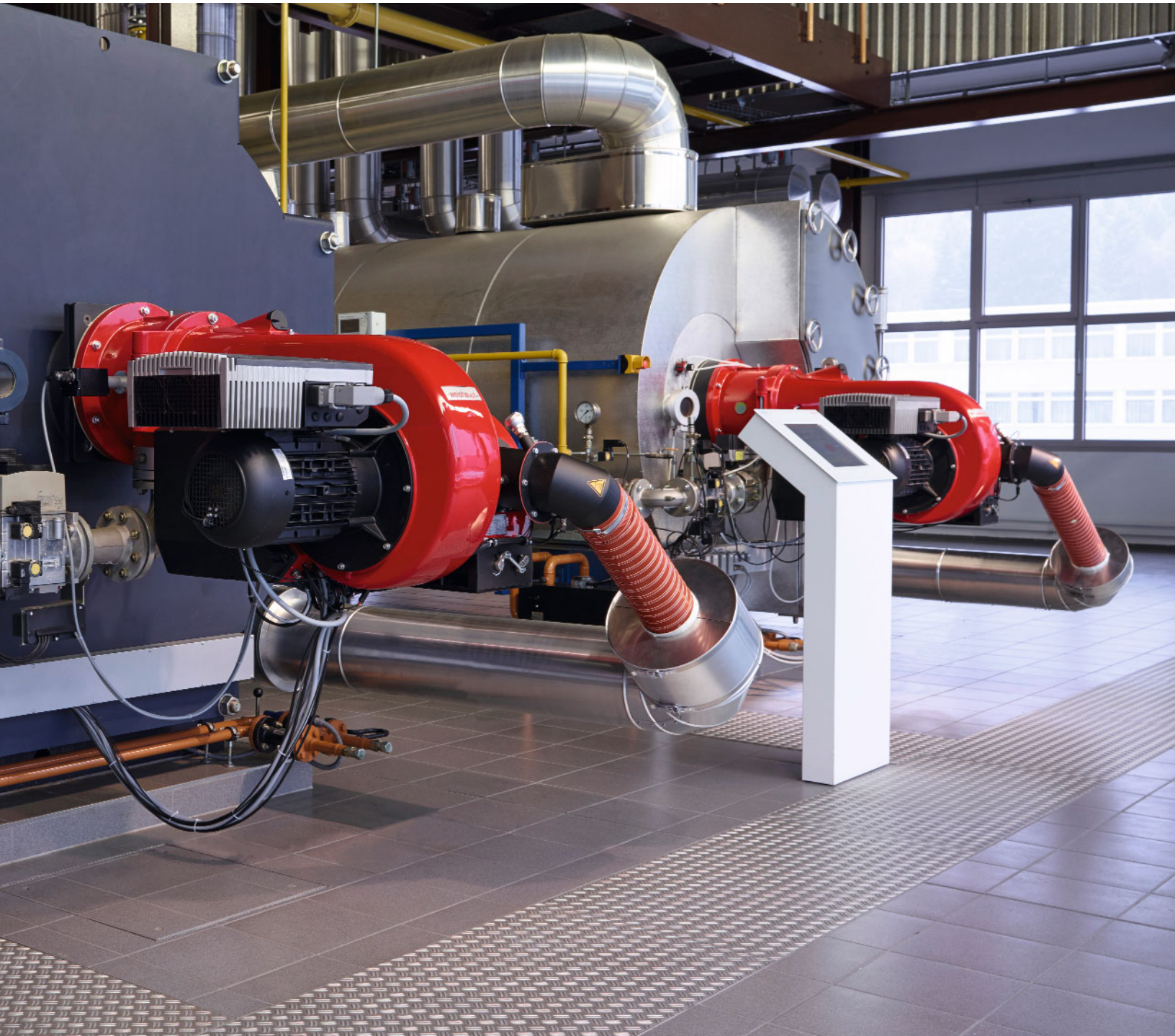
Burners with FGR on long-term test at Weishaupt factory's boiler room
