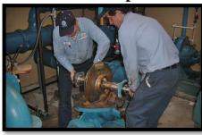
Our factory trained service technicians can handle most in-field applications ranging from on-site pump repair, pump removal, pump replacement, and general diagnostics.
