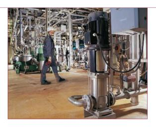
materials to bring you the best possible solution. This means that we can equip CR pumps with a shaft seal and bearing system that can withstand extreme heat and friction for longer periods of time. This makes them less unforgiving if the pump does run dry.
